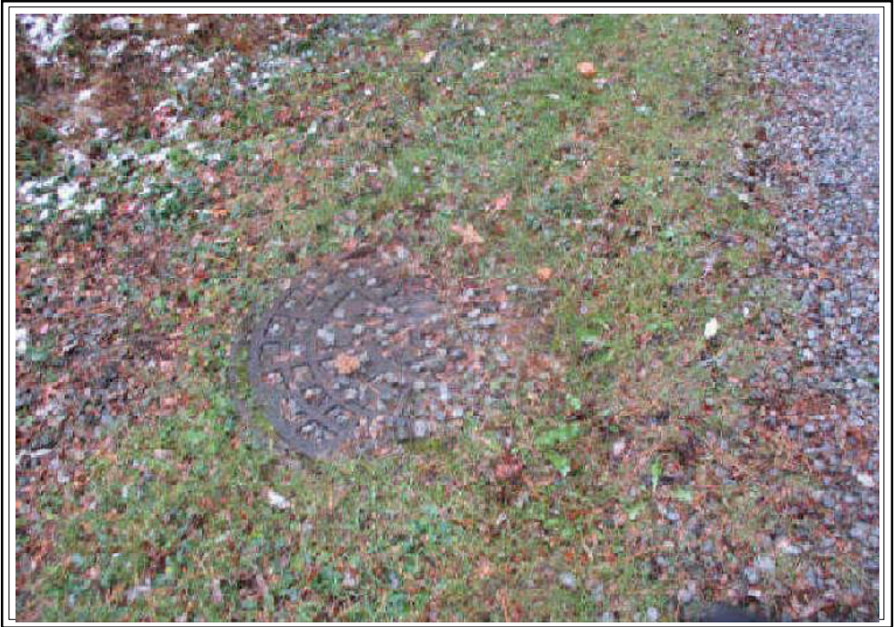
Sewer Man Hole Cover
